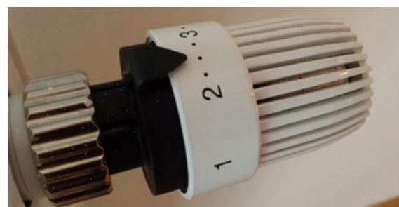
(88) Termostatski ventil.
