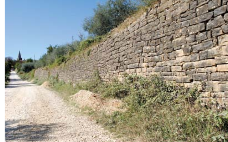
Figure 2: Dry stone retaining wall among a side road to Grožnjan (photo: Tanja Plešivčnik)
