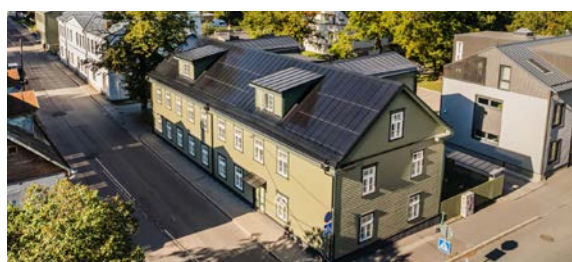
(88, 89) FN-moduli v videzu pločevinaste kritine (vir: Roofit)
