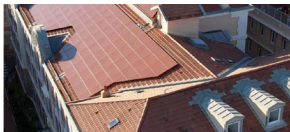
(86, 87) FN-moduli BISOL Spectrum v barvi kritine (vir: BISOL)
